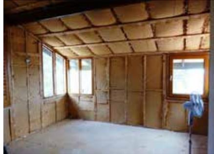
*Internal compressed wood fibre pulp insulation – Photo courtesy of building owner*
